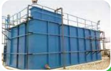
Membrane bioreactor at a construction company
