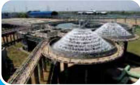
Cascade aeration at a power plant
