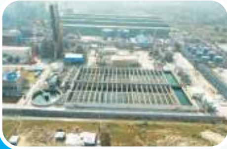
Effluent treatment plant at a steel industry
