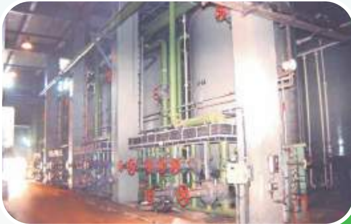
Softener at a power plant
