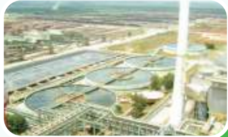
Clarifiers section at a paper plant
