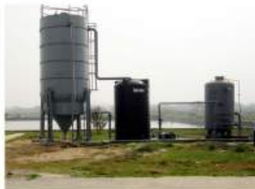
Continuous Sand Filter for Surface Water Treatment
