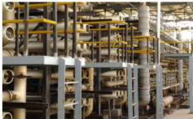
Sea Water Reverse Osmosis (Desalination) at Thermal Power Station
