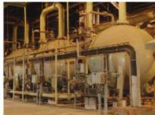
Condensate Polishing Units for Power Plant
