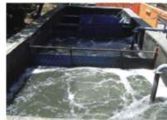
Fluidised Media Reactor for Sewage Treatment & Water Recycle
