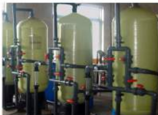
Arsenic Removal Plant for Ground Water Treatment
