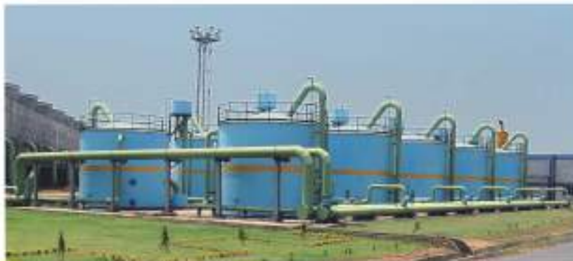
Side Stream Filters at Steel Facility
