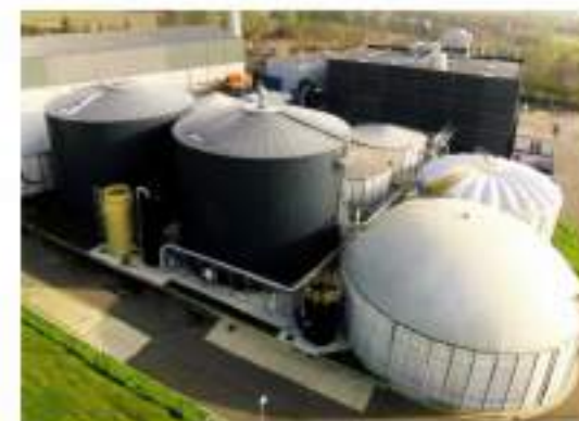
Sludge Digestion - Waste-to-Energy
