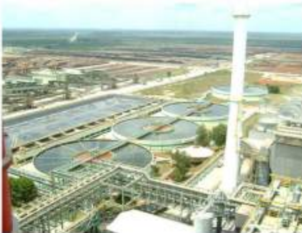
High Rate Solid Contact Clarifiers for Paper Industry
